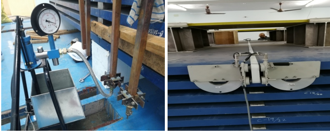
(c) Hydraulic testing of brazed joint.
