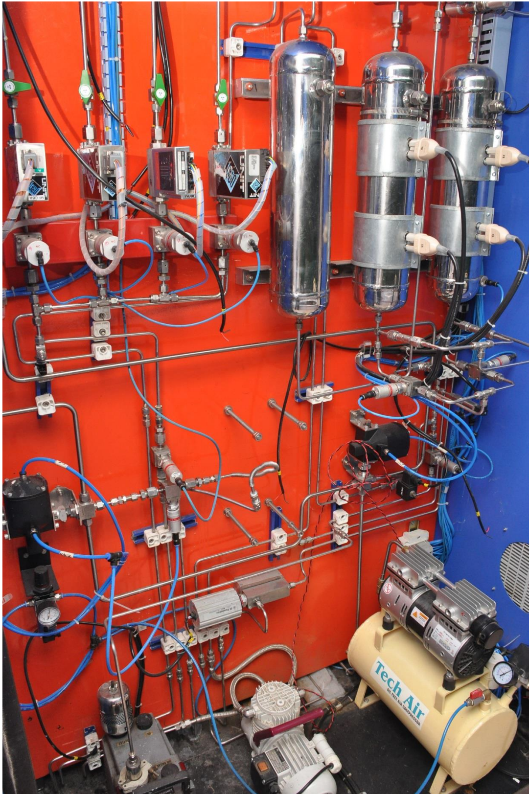
Photo-sheet of Closed Loop System (Rear View)
