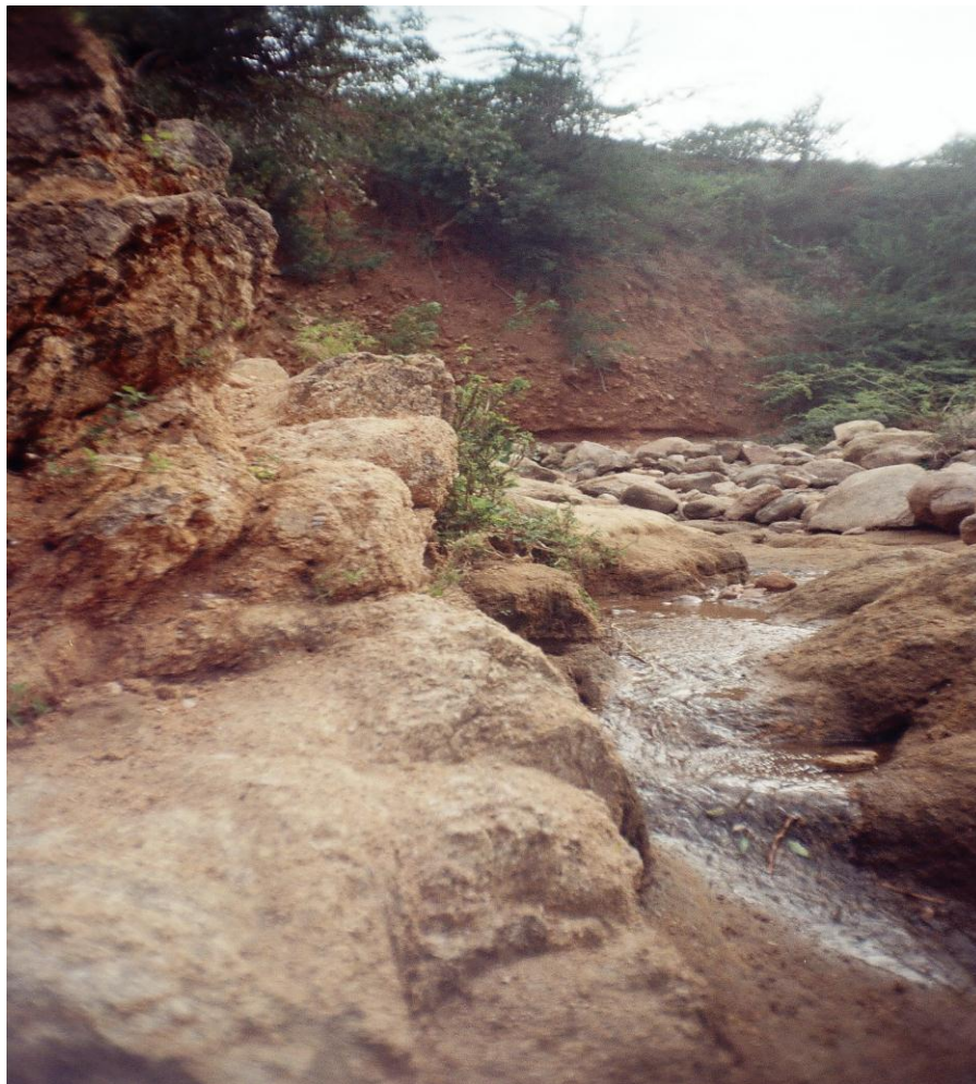
Figure 4.4 Stream at the INO site - Box culvert to be constructed
