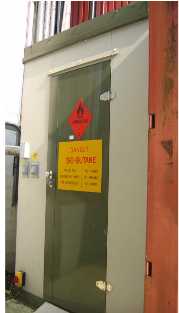
Special room for Iso-butane and R134a gases
