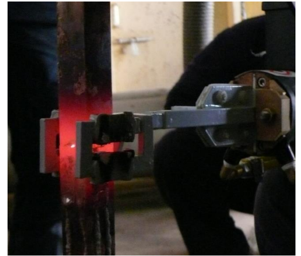
Induction brazing in progress
