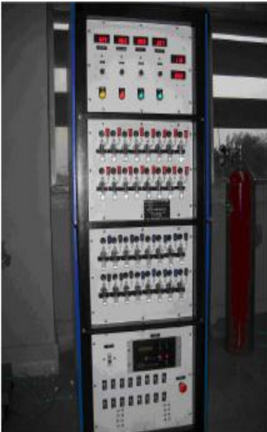
Gas mixing unit
