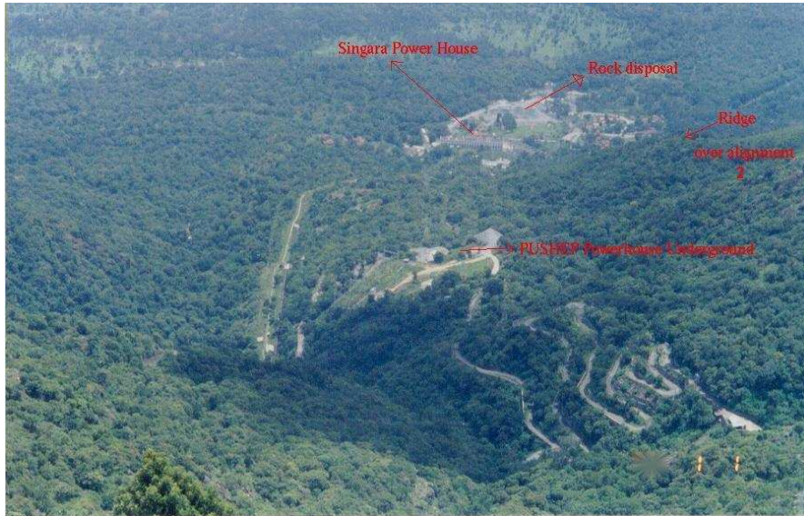
Figure 4.1: A View of PUSHEP location from Glenmorgan.
