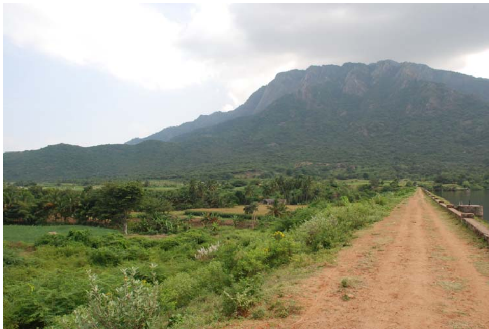
View of the Pannapati Dam with, at the bottom of the hill; a site assessed for the tunnel portal.
